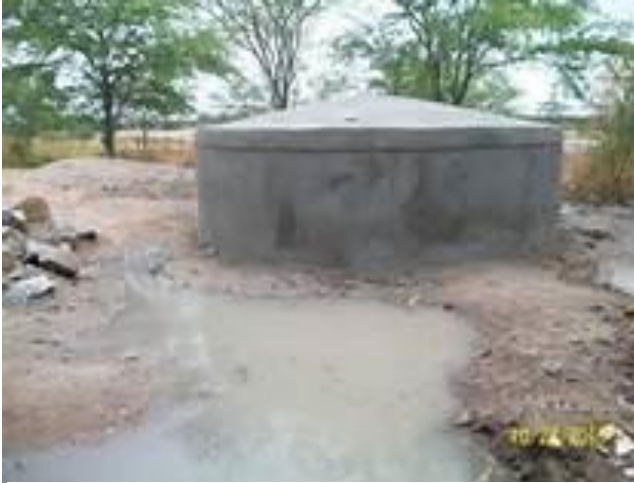
Ferro Cement Tank
