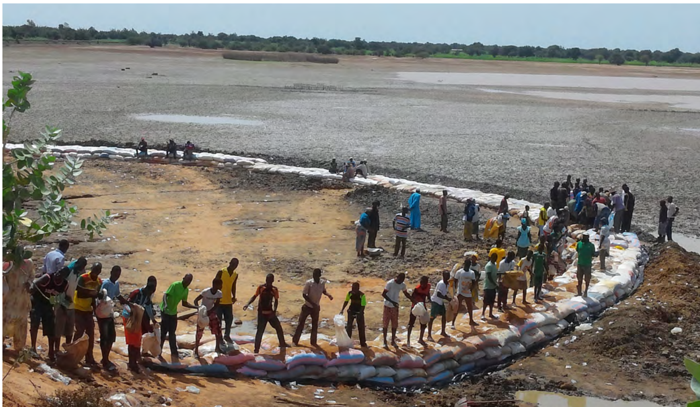
The community is mobilised for the reconstruction of the dyke.
